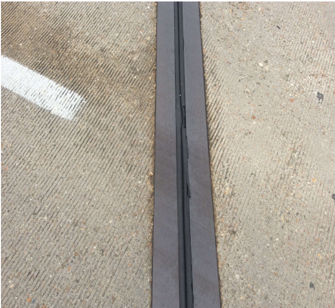
PHOTO 2 Description Bent 2 north bound joints seal torn and leaking
