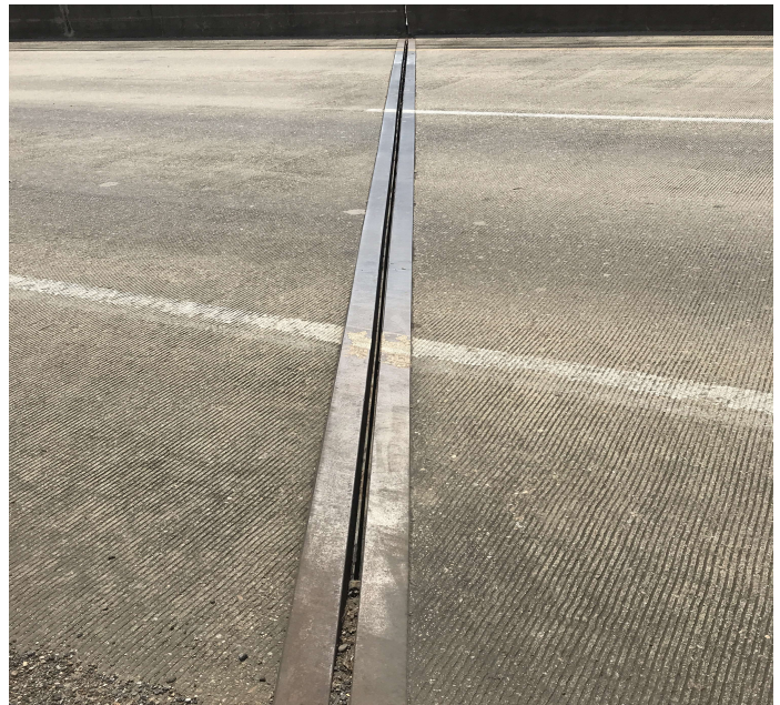
PHOTO 1 Description Joint - Bent 2 Pile 3 Left: Loss of adhesion
