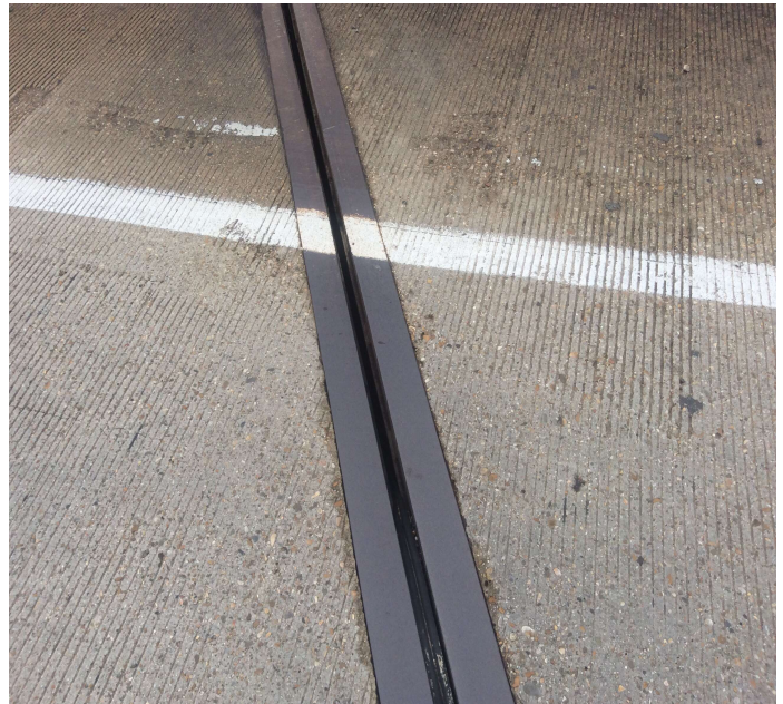
PHOTO 4 Description Bent 3 south bound joint seal missing and leaking
