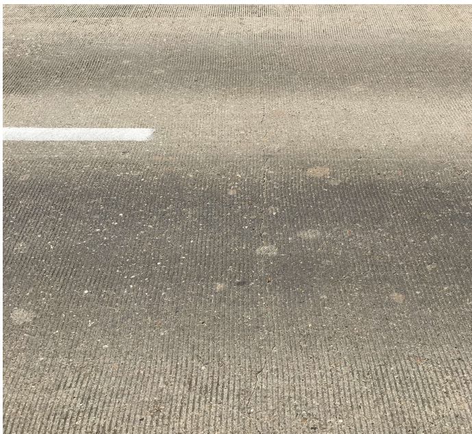
PHOTO 2 Description Deck - Span 3 : Cracking
