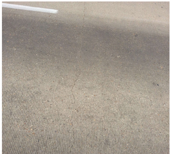
PHOTO 1 Description Span 4 north bound transversely cracking on deck
