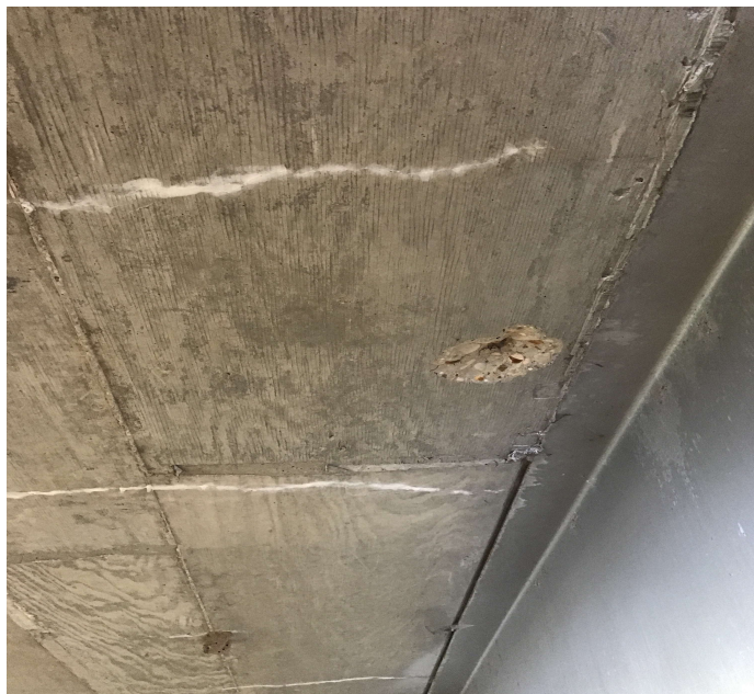
PHOTO 3 Description Soffit - Span 3 Bay 5: Spall and reflective efflorescence
