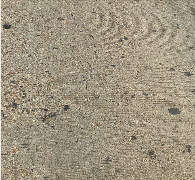
PHOTO 5 Description Deck - Span 2 right: Cracking
