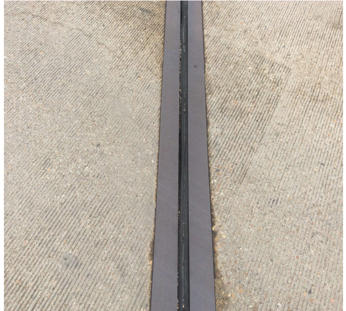
PHOTO 3 Description Bent 3 north bound joints seals lose of adhesion and leaking
