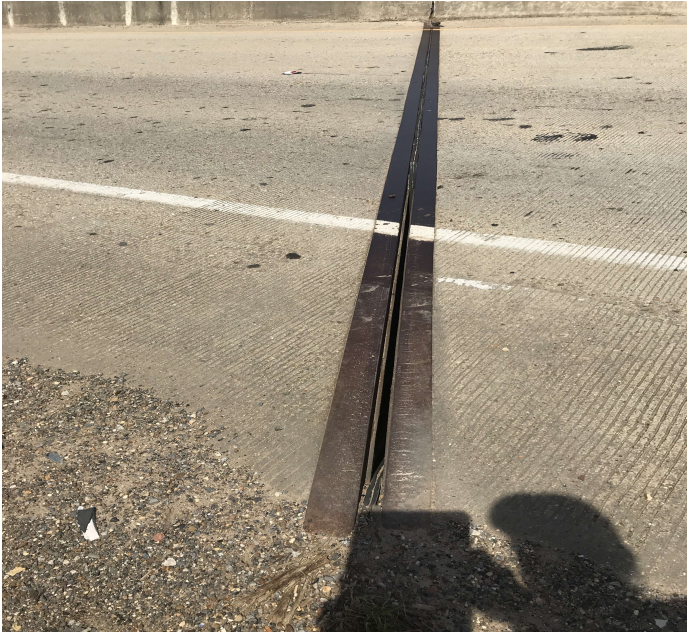
PHOTO 2 Description Joint - Bent 3 right : Loss of adhesion
