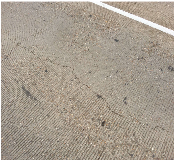
PHOTO 2 Description Span 2 south bound longitudinal and vertical cracking on deck but common on north bound also
