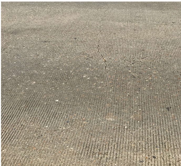
PHOTO 1 Description Deck - Span 2 : Cracking
